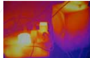
Power outlets and surge suppressor.
